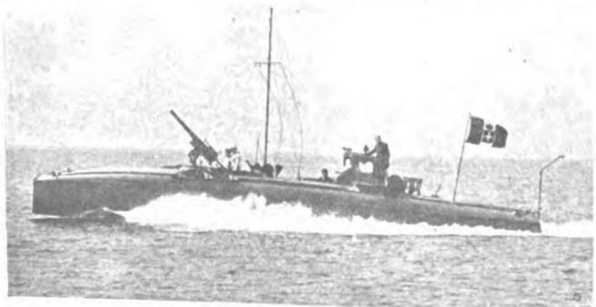
Sub-chaser Used by Italian Government These were built by Gio Ansaldo & Co. of Genoa, Italy, and were powered with motors built by the Sterling Gas Engine Co., Buffalo.
