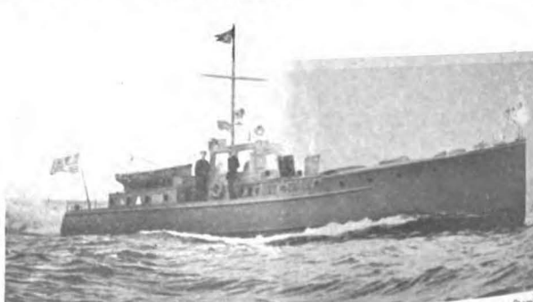
Type of Private Yacht Used by America for Patrol Service A 71 footer turned over to the government by Ralph Pulitzer. She was powered with two 8-cylinder Duesenbergs. Speed, 25 miles.
